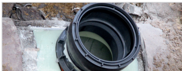
Built-in Pipe Liner Lateral Connection System Connex
